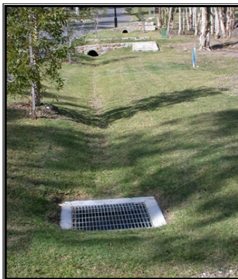
PLATE 8.2 – TYPICAL SWALE
